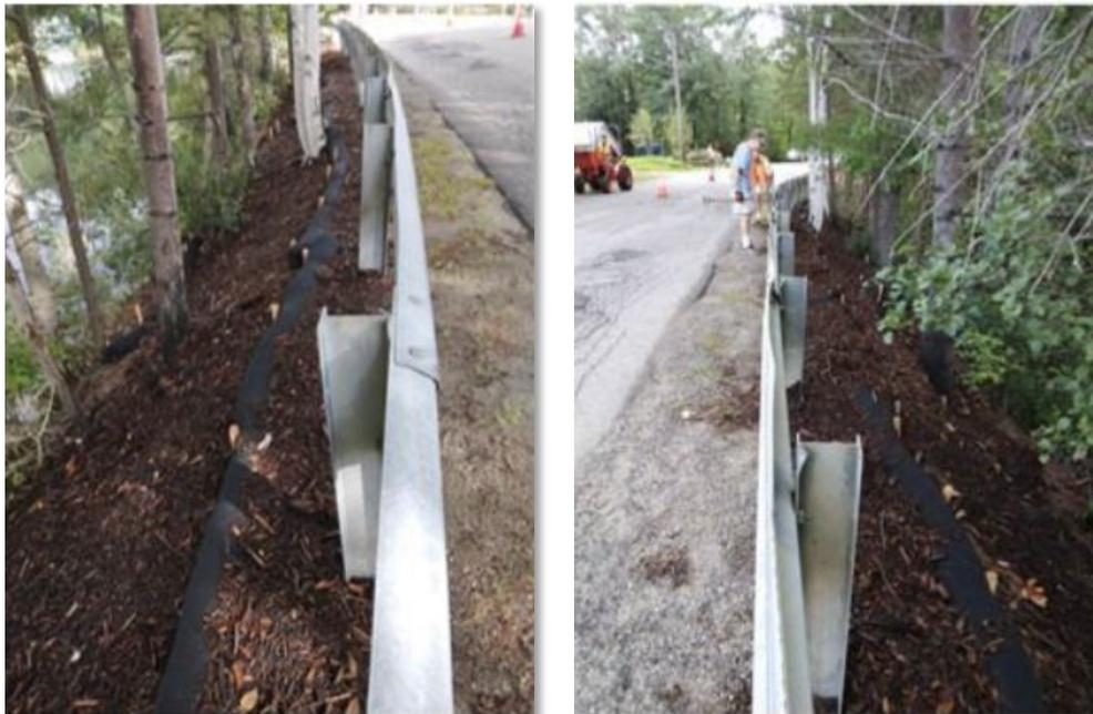
Site #1-14 just south of the culvert crossing shown above. West side is shown on the left and East side is shown on right. Both photos demonstrate the after condition. Note terracing ECM and staked ECM filled socks.
