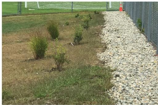
After – A drip edge filter with riprap was installed to slow and filter runoff from the tennis courts. Eroding slope was regraded and planted (looking across top of slope).
