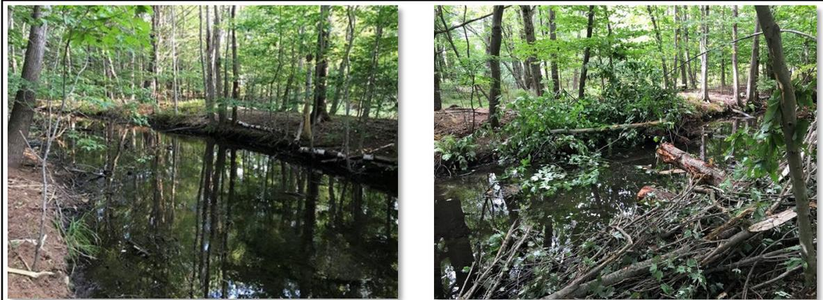
Woody debris installed at the Seneca Ave site. Before photo (left) shows an artificially straightened stream with stagnant flows and low levels of dissolved oxygen. After photo (right) shows conditions after addition of woody debris.
